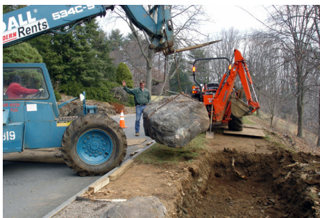
Largest rock element being placed— about 6,000 pounds. (March, 2008)
