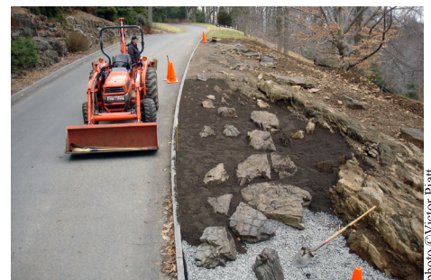
Scree medium being laid. (February, 2008)
